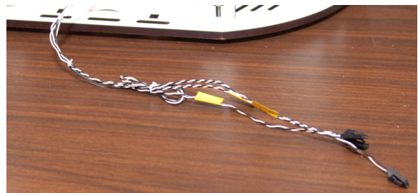
Fig. 17.3-4: Finished end-stop wiring.
